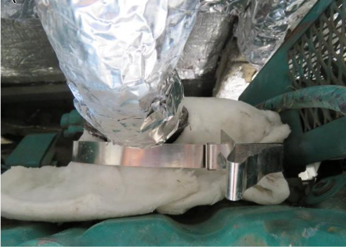
Bottom view after manifold is wrapped and strapped.
