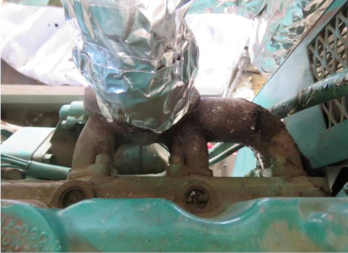
After exhaust pipe was wrapped and before manifold is wrapped.
