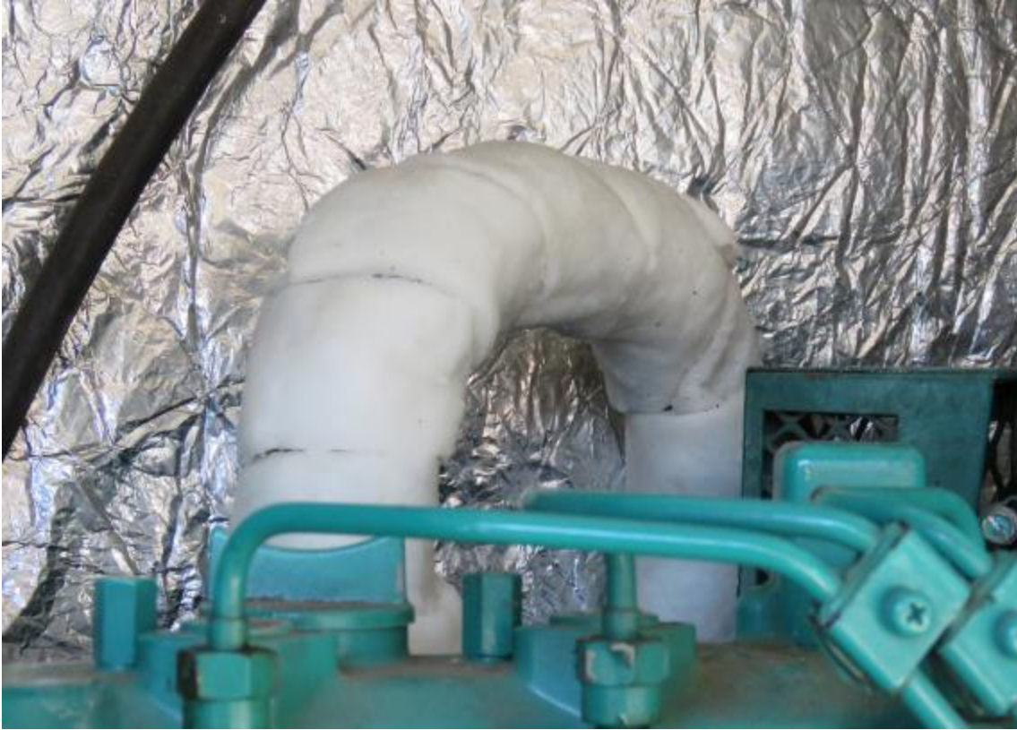
Generator with the ceramic Wet Blanket wrap installed before it sets up.
