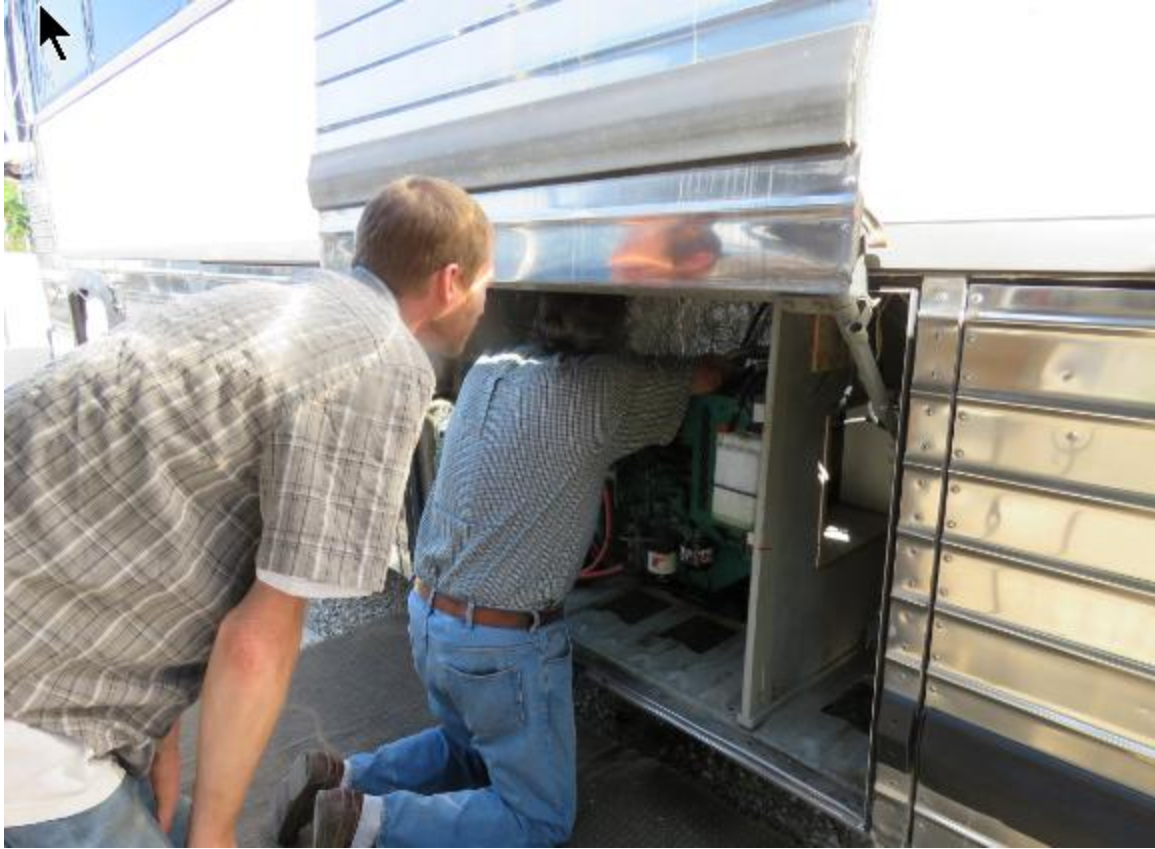
Penn installing the insulation as Todd observes.
